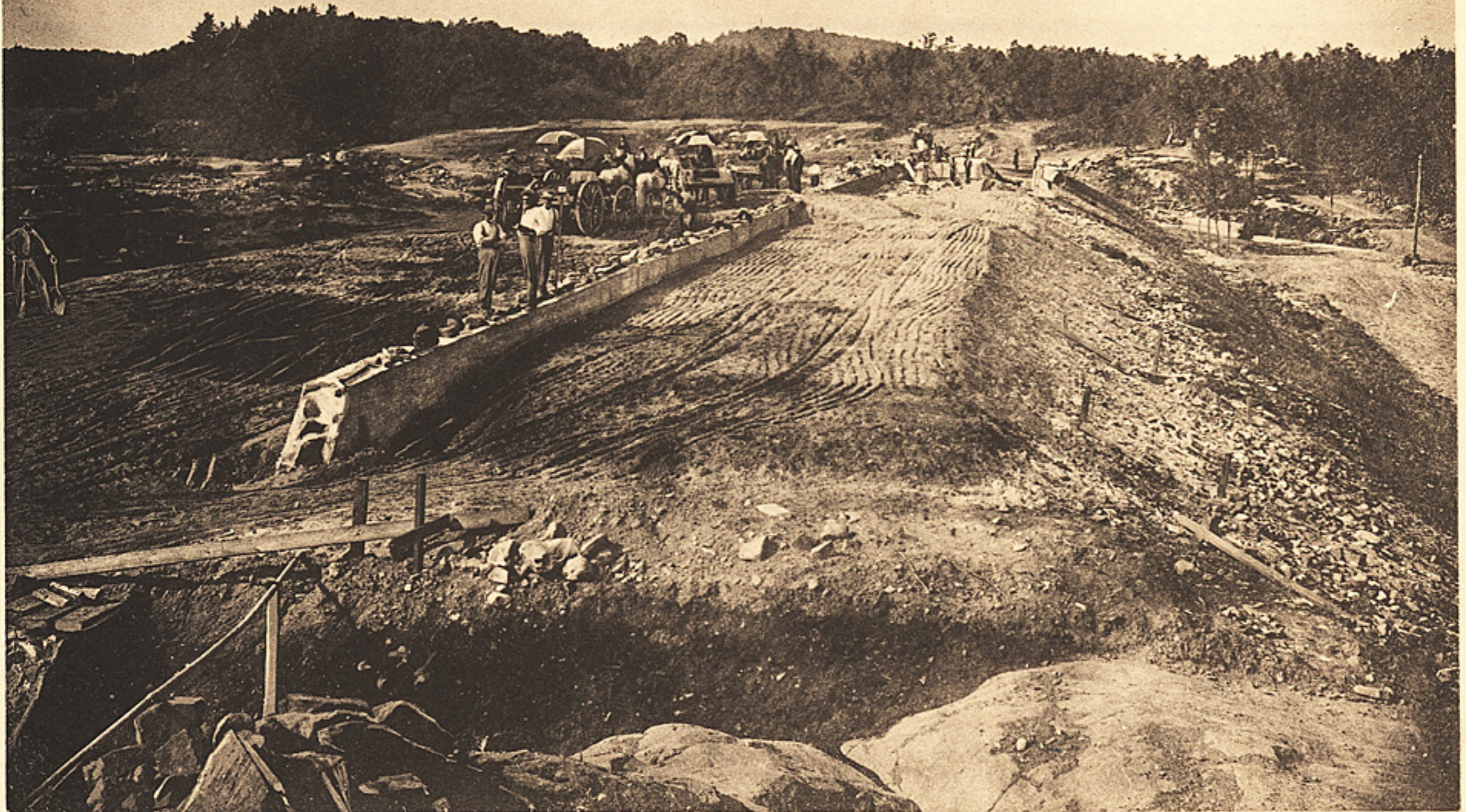
HIGH SERVICE RESERVOIR. Showing dam nearing completion. July, 1904.
